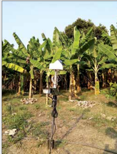
Continuous profile soil moisture sensor installed in the Attappadi CZO
