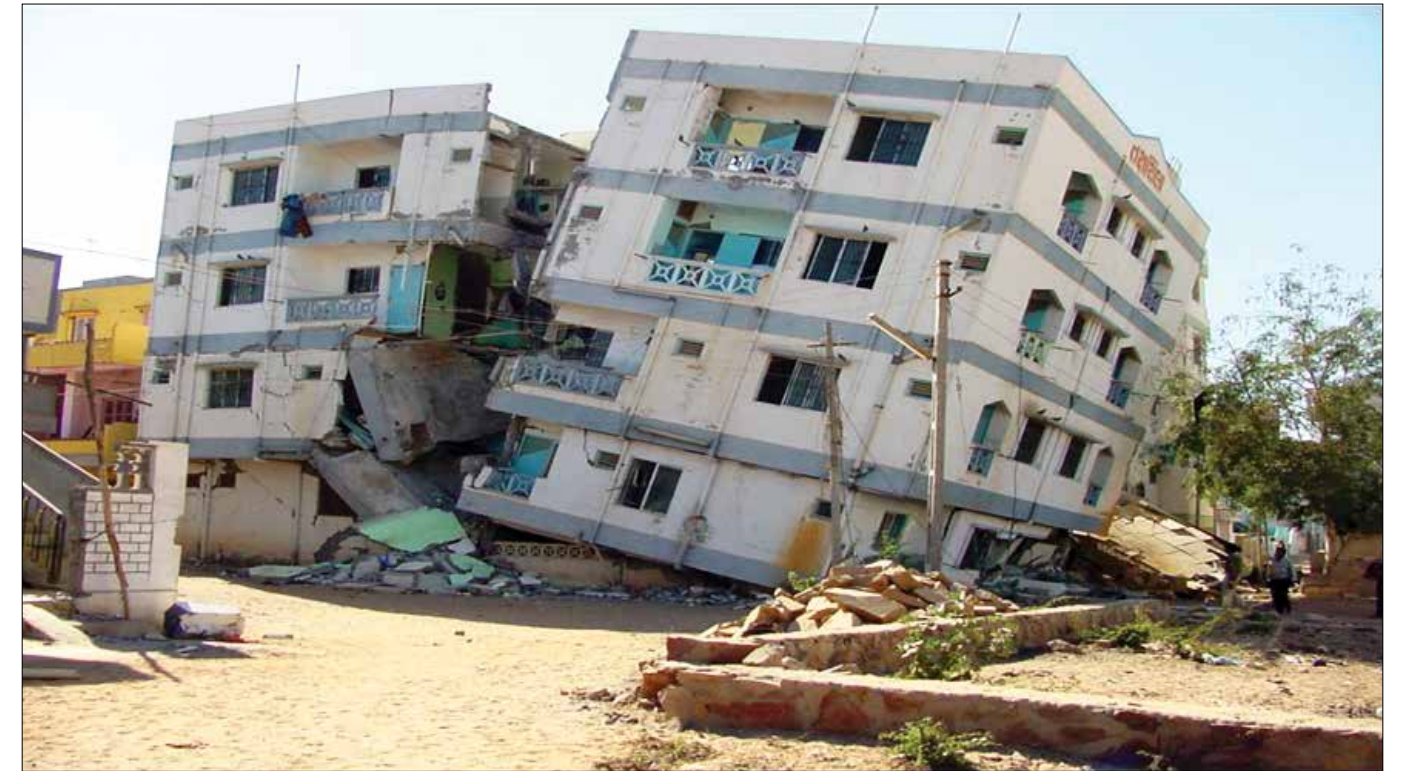
Damage to buildings after the Bhuj earthquake of 2001
