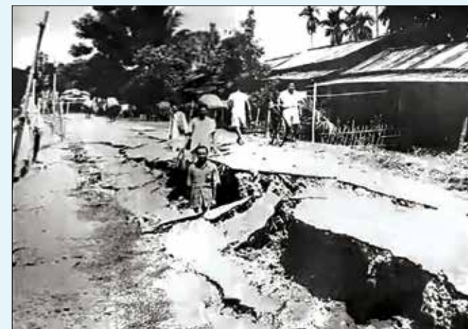
Damages to road and bridge during 1950 Assam earthquake
