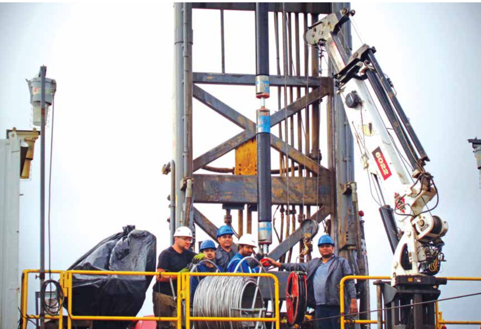
Lowering of a double straddle packer system into the pilot borehole for hydrofrac tests
